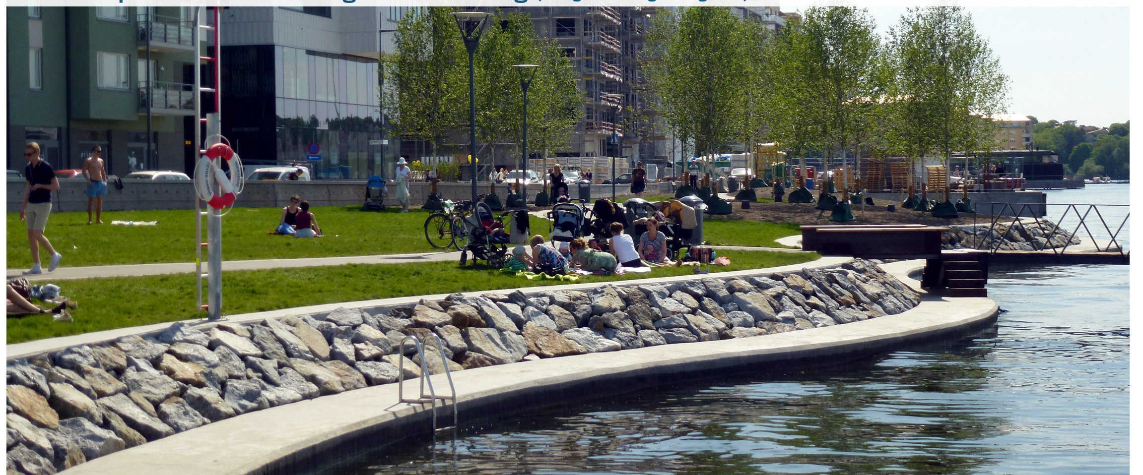
Example: Hornsbergs Strandpark, Sweden. A linear park that addresses the waterfront and is a passive defence against flooding (Image: © Holger Ellgaard)
